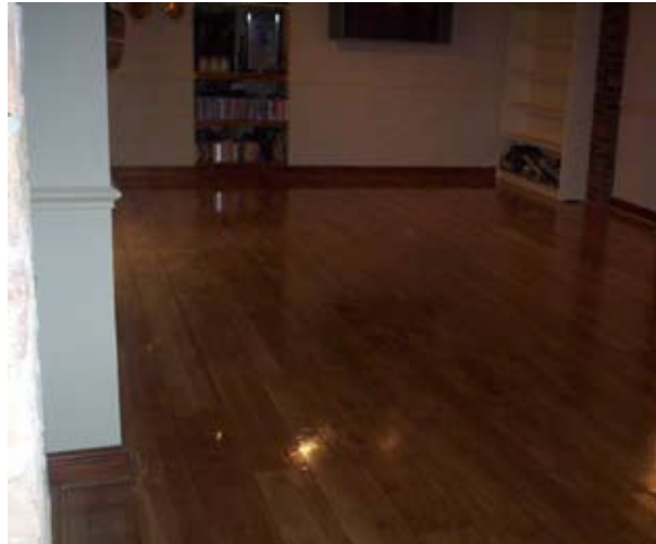
Wood floor after sealer and finish coats applied
