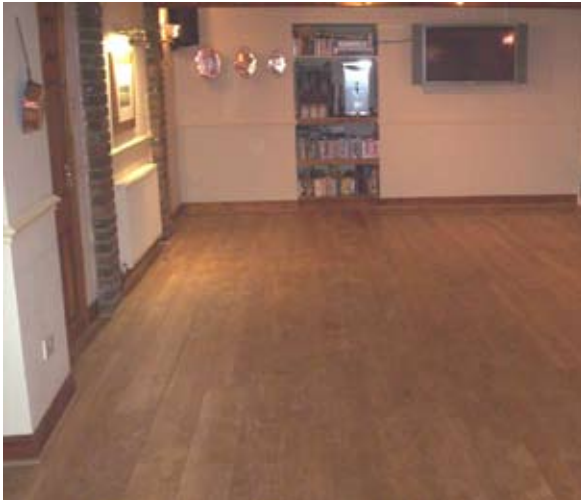
Wood floor after sanding B4 finish applied
